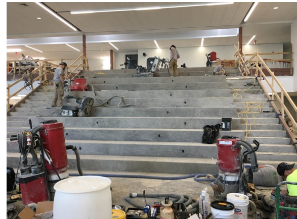
Social Stair – Concrete Polishing
