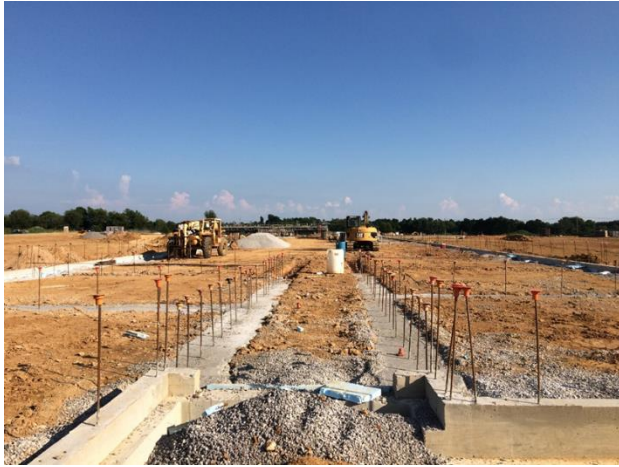
Interior Foundations (E)
